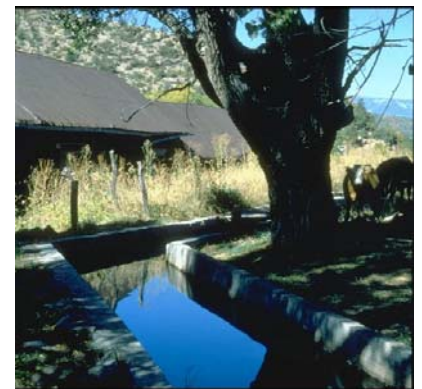
Fig. 1.2: Concrete-lined channel. Stream systems across the nation have been altered for a wide variety of purposes.
