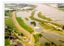
View on side channel set of Floodplain "Gameren", downstream direction. Photo: Rijkswaterstaat (NL)
